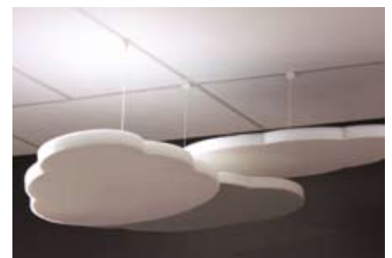
Absorbents figure-sawed as clouds. Size 1000x700x50 mm.
